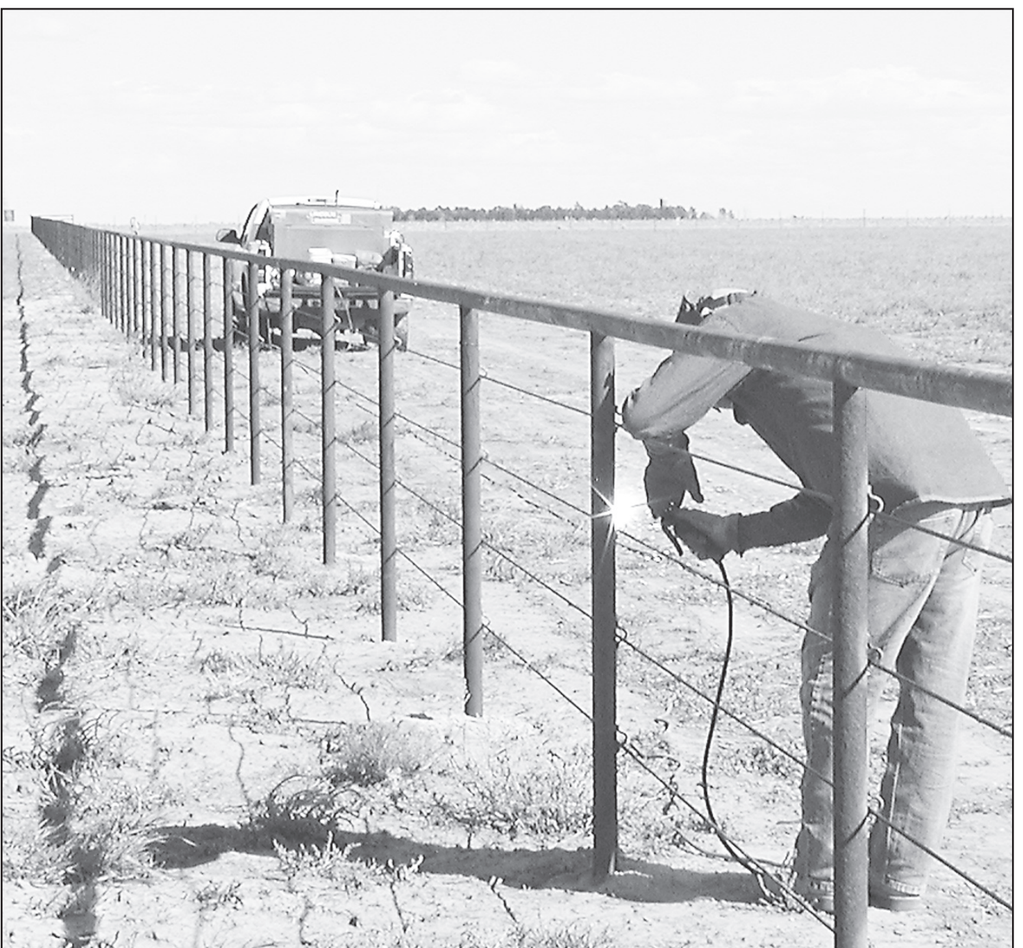
LOTS GOING ON AT THE DAIRY — A worker welds fence at the Bird City Dairy.
