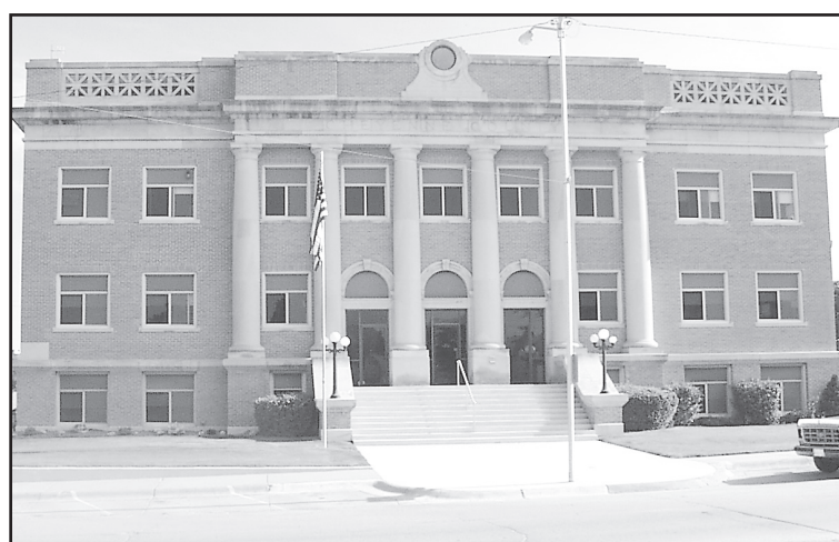
Cheyenne County Courthouse
