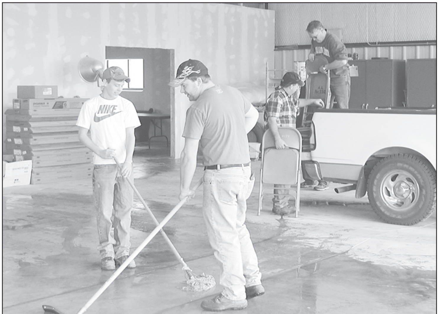
GETTING READY for company. (l to r) Jeremiah, Lucius and Loren White, and Gary Brubaker clean up the Egger's Emergency Building for the hamburger fund raiser to be held there. The new addition in the facility will be used as a medical training room.
