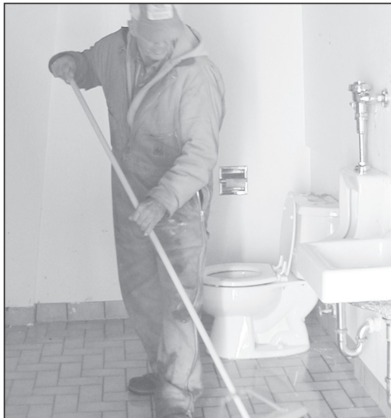
FLOODING FROM BROKEN WATER PIPES causes major flooding in the Wesleyan Church. With nearly 2 inches of water in some areas, Dick Bursch is busy moving water to the front entrance.
