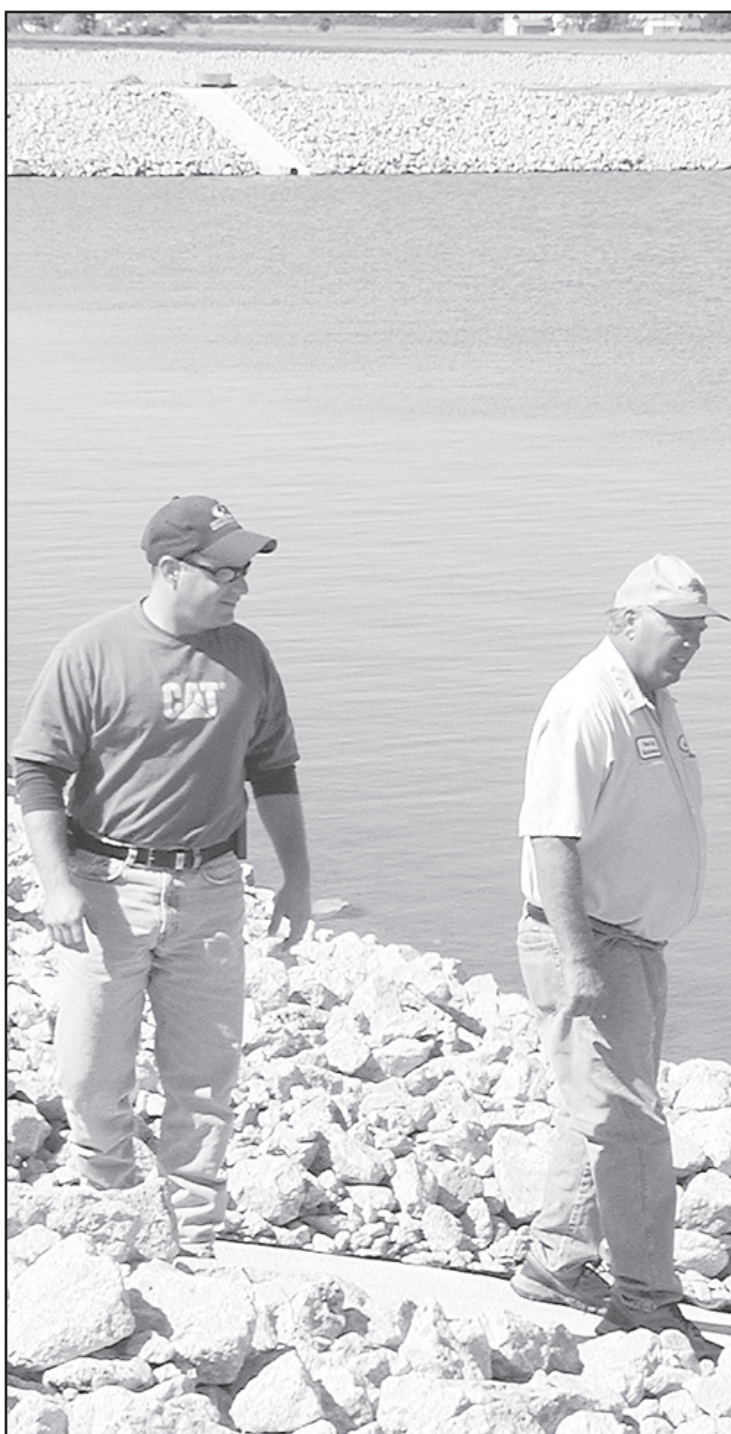
CITY MAINTENANCE WORKERS, Craig White, left, and Brad Schneider inspect the new wastewater lagoon. Times staff photo by Linda Schneider
