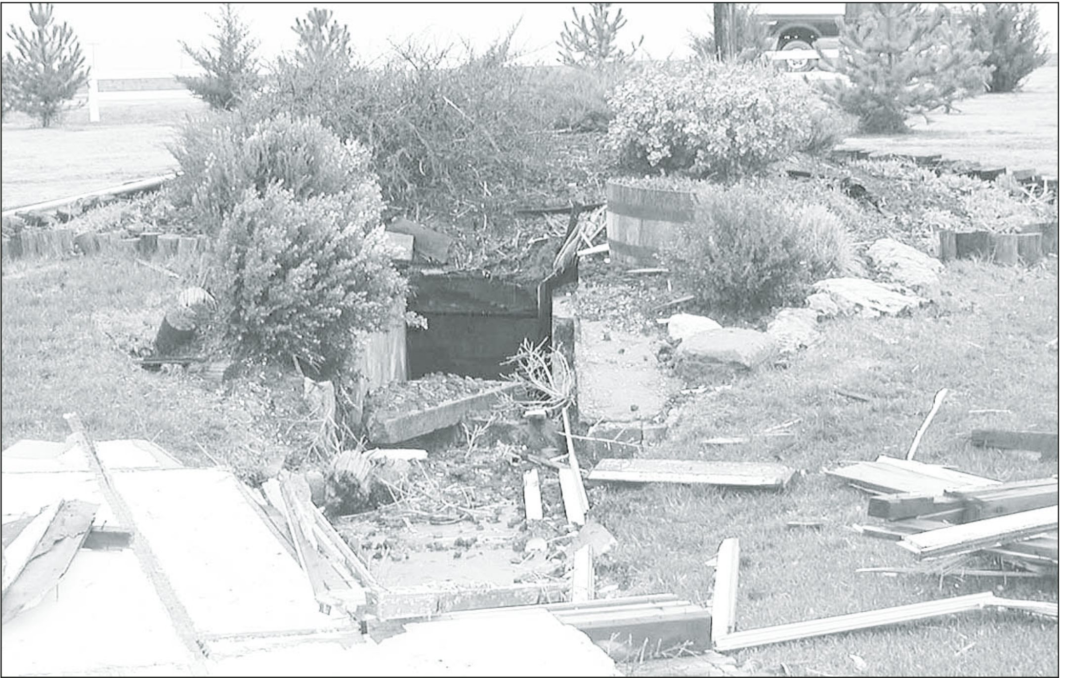
The cellar at the Nick Ketzner farm was a lifesaving place during the storm. However, the door was ripped off and a wagon wheel was thrown down the steps.
