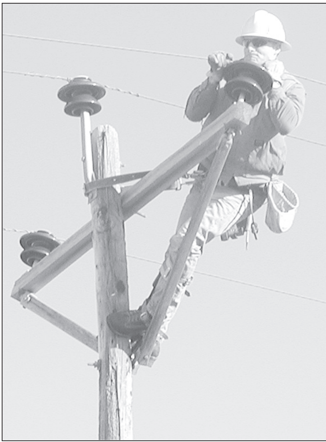
LINEMAN MARSHALL HESPE removes three lines from a pole that will be replaced. Winter months do not offer a break for a lineman. Times staff photo by Casey McCormick
