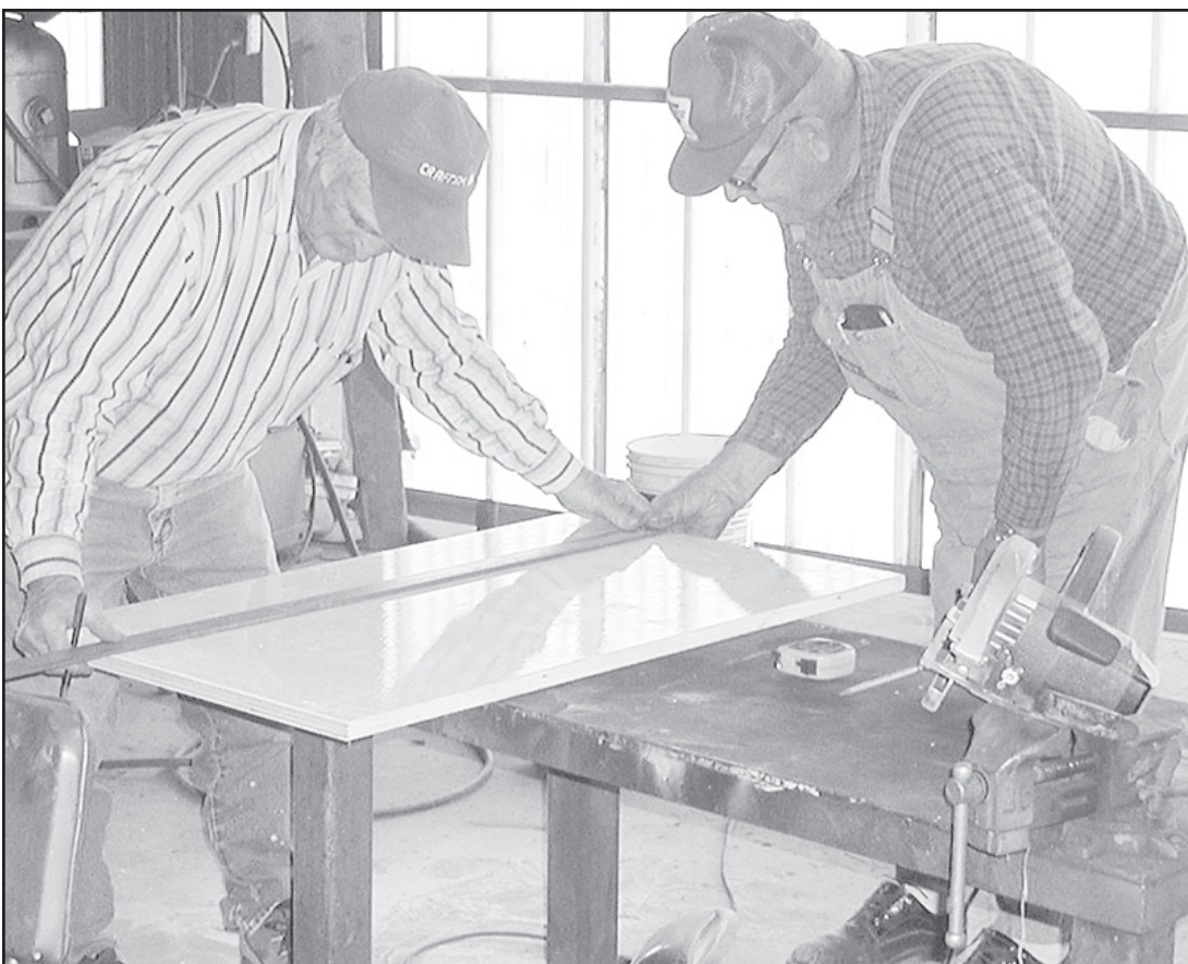
THRESHER SHOW —Larry Henry and Norman Dorsch are still keeping busy at the Thresher Show Grounds. The two men are building a box for a tractor.
